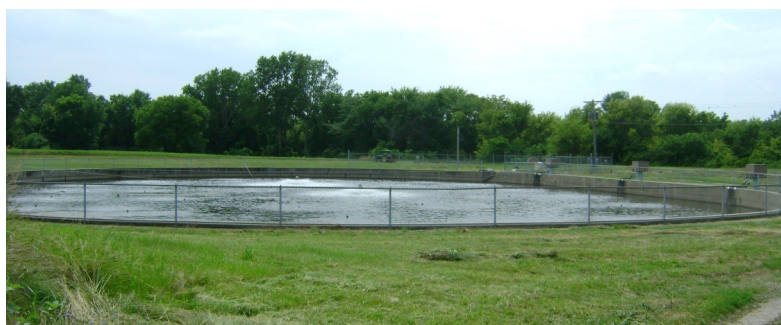
Typical wastewater lagoon
