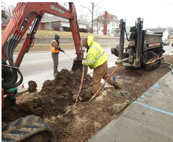
Installing broadband cables in Maryville
