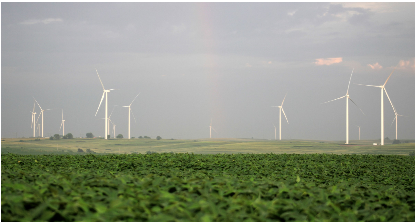
Atchison County Wind Farm
