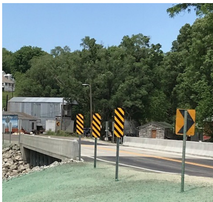
Mound City bridge replacement.
