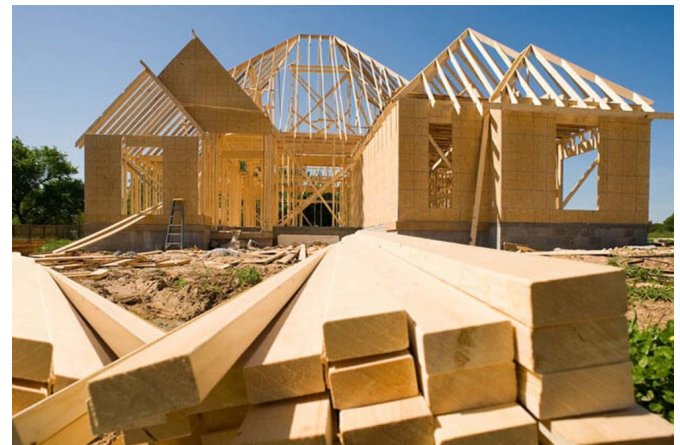
Single family housing construction.
