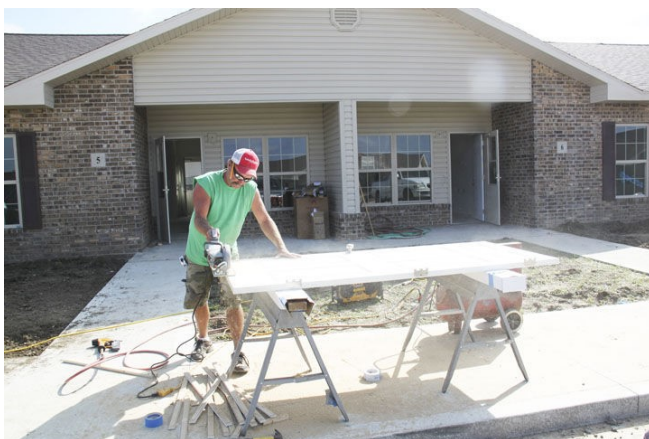
Multi-family units being constructed.
