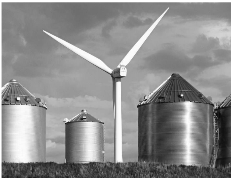
Clean energy provides economic opportunities across the northwest Missouri region.
